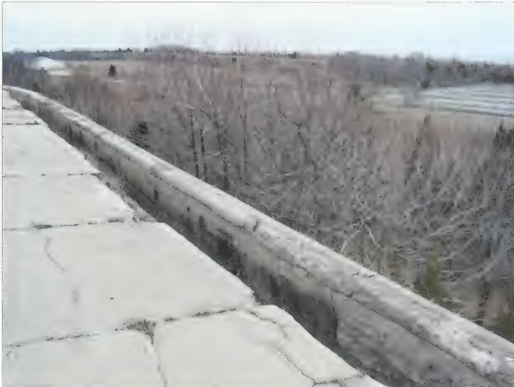
Figure 3.26. View looking north across chemin de ronde , Battery Potter. The superior slope gently descends to a sentry route known as a chemin de ronde that is fronted by a parapet wall (Olmsted Center, April 2008).
